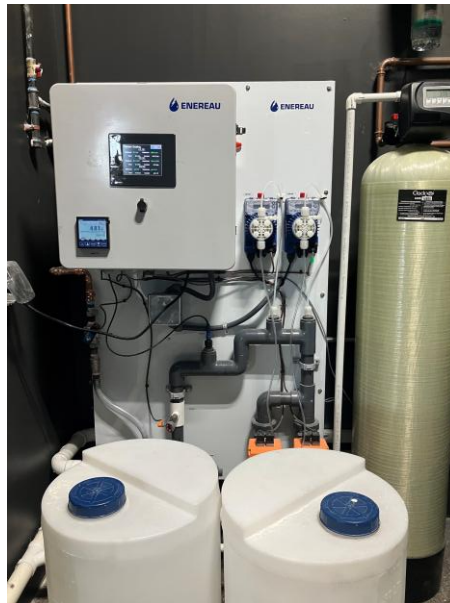
Skid mounted pH system regulates wastewater and controls discharge to drain only when in acceptable range (pH 6-8)
